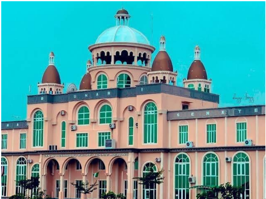
Senate Building of Northwest University, Kano, one of the two State Universities established in Kano by RMK
